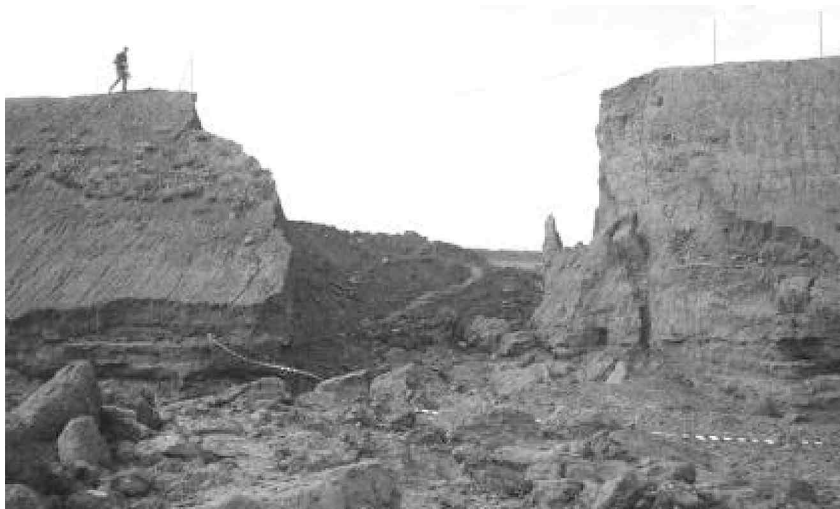
Figura 3. Vista general de la rotura de la balsa de San Juan (Altorricón, Huesca) Figure 3. General view of the San Juan Dam break (Altorricón, Huesca)
