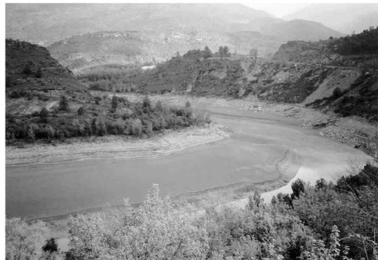
Figure 5. Above, silt (76%) and clay (19%) sedimentation in the Barasona reservoir (Ésera and Isábena Rivers, Ebro basin). Below, sedimentation in the Camarasa reservoir (Noguera Pallaresa River) (photographs by the author, April and June, 2001).
