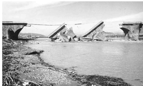
Figure 15. The Carlos III bridge (XVIII century) in the Llobregat River after its collapse during a flood in 1971. Lack of sediment feeding from upstream due to gravel mining was the main cause.
