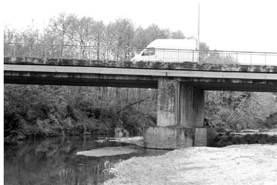
Figure 14. The N-II road bridge in the Lower Tordera (above) and the A-7 access road bridge in the Tordera near Hostalric (below) illustrate river-bed incision due to gravel mining from the fifties (photographs by the author, June 2001).
