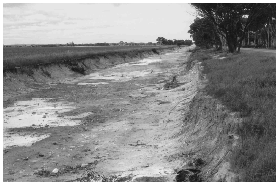
Figure 16. Drain excavated to evacuate saline groundwater and lower the water table, near Corrigin, southwest of Western Australia.
